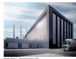
Hinkley Point C - Proposed Turbine Hall
