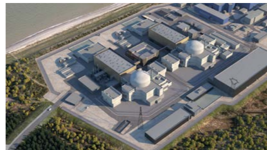
UK EPR™ Safety Related Buildings aerial view
