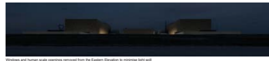
Windows and human scale openings removed from the Eastern Elevation to minimise light spill
