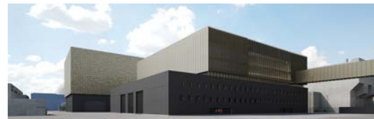
View of Eastern Elevation to the Operational Service Centre within the context of the Turbine Halls
