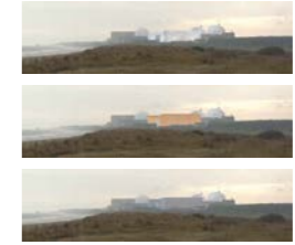
Prominent Facades of Turbine Halls viewed from the north - colour in the landscape
